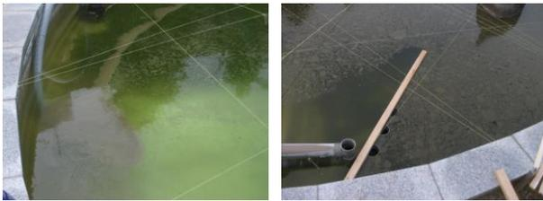
図3 Appearance of floating sludge immediately after stirring, sludge removal by overflow
